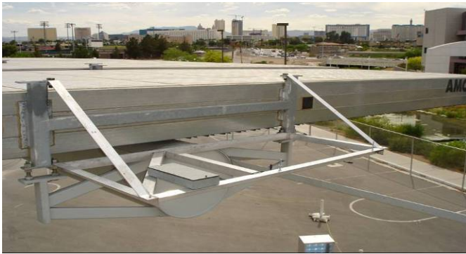
Figure 4-3. Mounting frame bolted to weldment.
