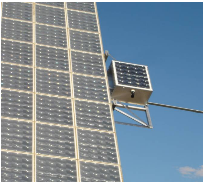
Figure 4-4. Multi-junction module on the UNLV HCPV system.
